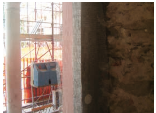
BELGIRATE: villa Matilde castle, correction of thermal bridges of doors and windows.
