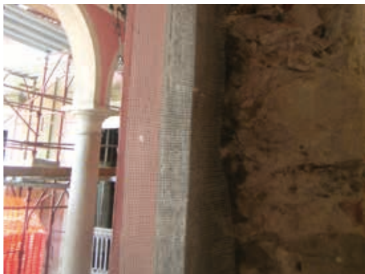
BELGIRATE: villa Matilde castle, correction of thermal bridges of doors and windows.
