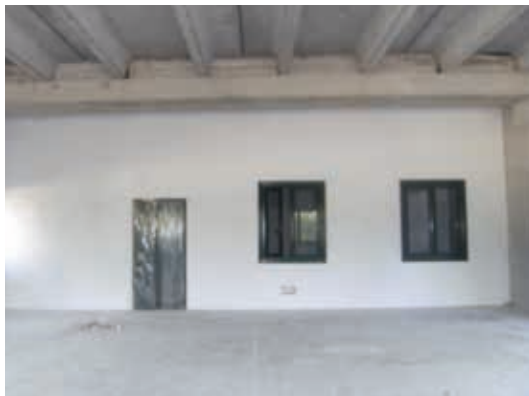
LODI: dividing walls for offices and canteen.
