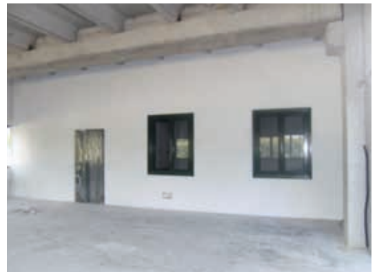
BELGIRATE: villa Matilde castle, correction of thermal bridges of doors and windows.
